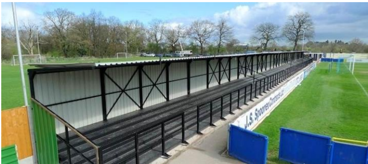
Drain Tech End
